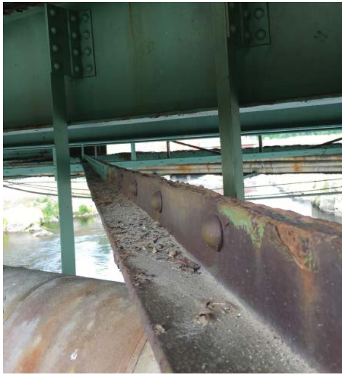
Photo #53: General top view of lateral bracing span from sidewalk truss to non-sidewalk truss in spans 1 & 2 (8/2/16)
