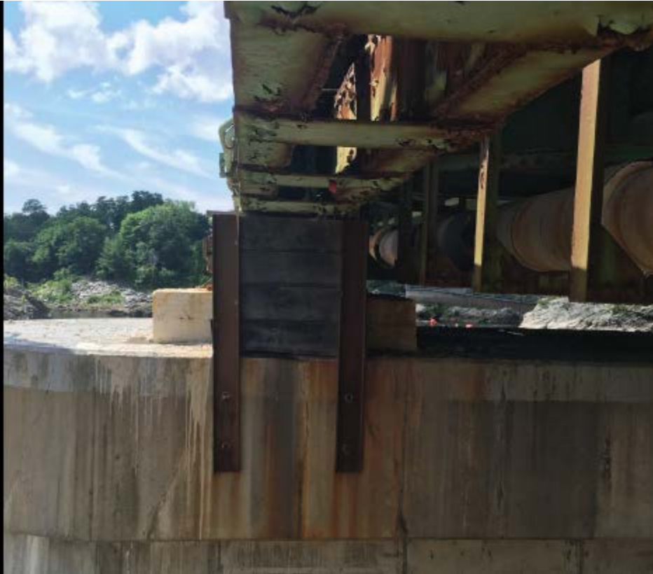
Photo #58: Shoring of non-sidewalk bearing, pier 2, span 3 (looking south) (8/2/16)
