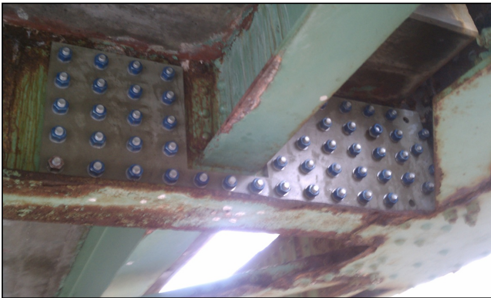
Photo A26 – End result of similar repair to Floorbeam.
