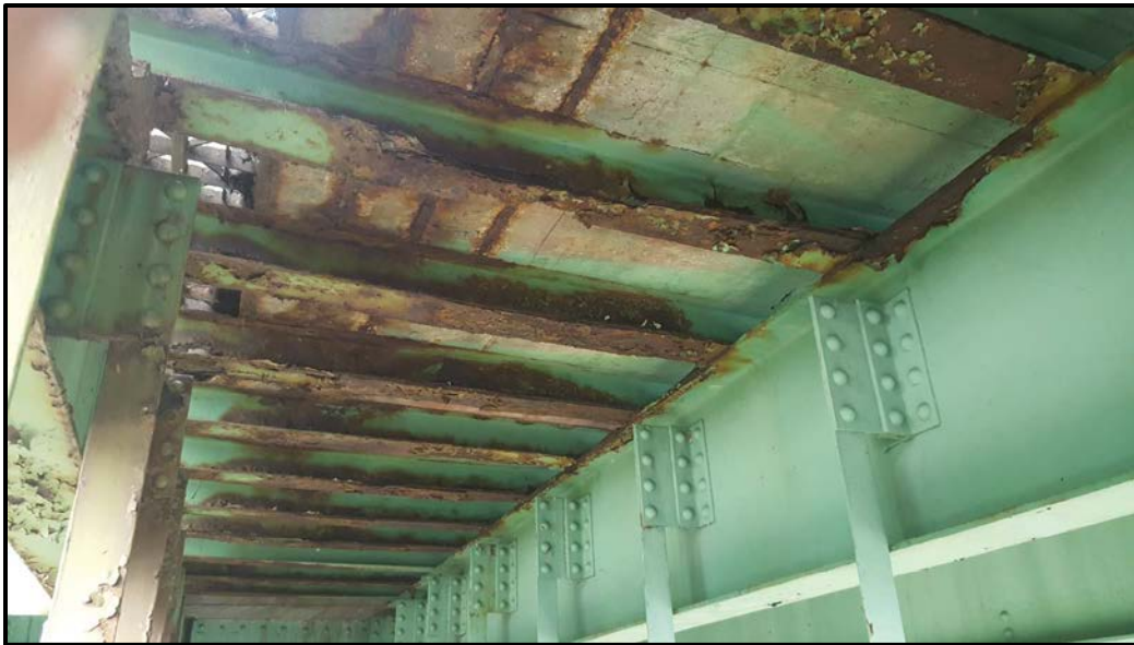
Photo A21 – View showing Needle Beams between Stringers 7 and 8. Area between stringers 3 and 4 are similar.
