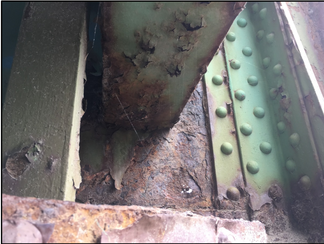
Photo A2 – Floorbeam 5, Roadway Truss @ Stringer 8 (Exterior)
