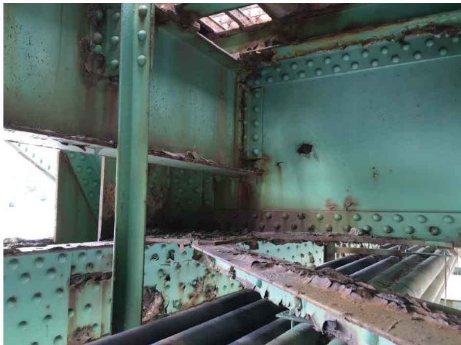
Photo #24: Typical exterior stringer (S3 & S8) to floor beam connection (Typ. all spans) (8/1/16)
