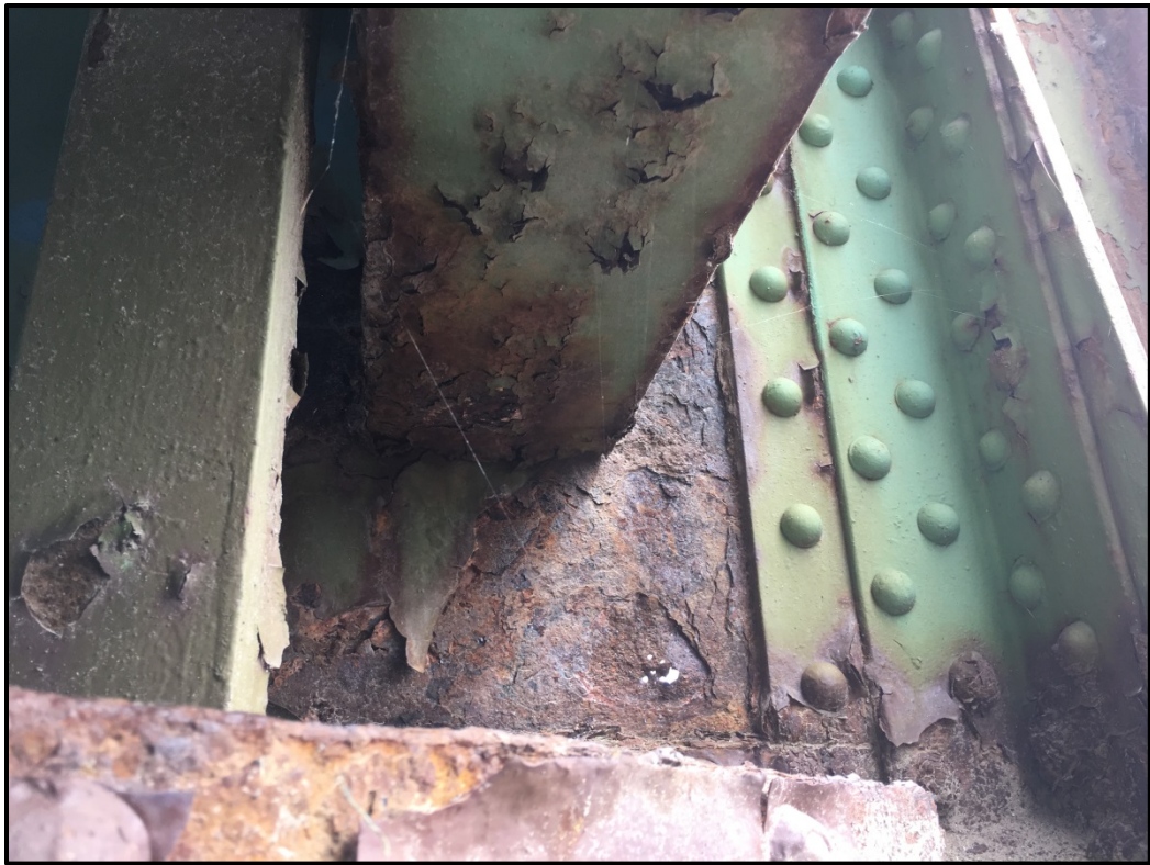
Photo A2 – Floorbeam 5, Roadway Truss @ Stringer 8 (Exterior)
