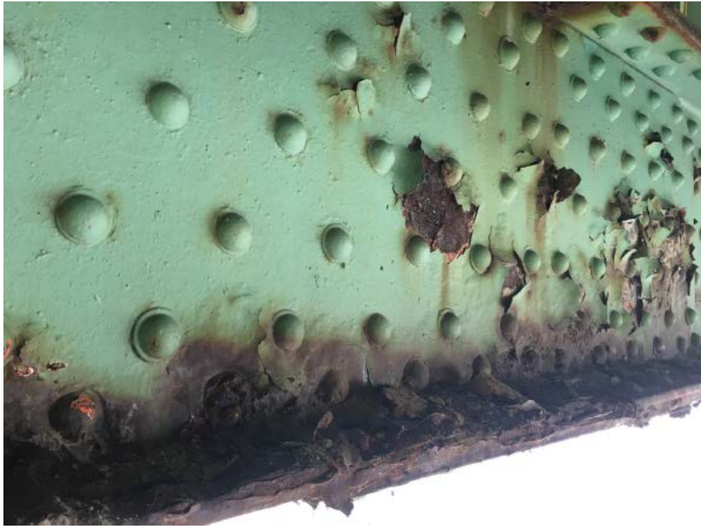
Photo #35: Bottom chord of non-sidewalk (eastern) truss, in span 1 near FB 2 (8/1/16)
