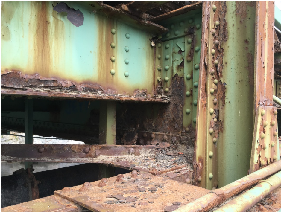
Photo #5: General view of the Floor Beam, Stringer & Vertical Truss member connection (8/1/16)
