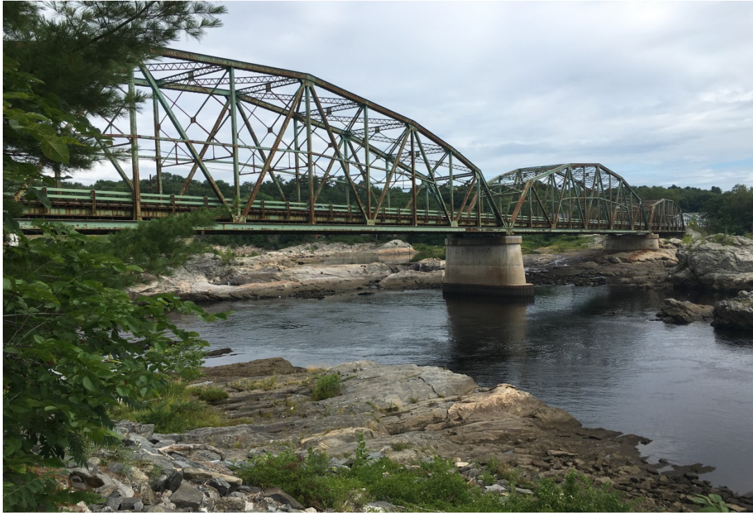
Photo #1: General view of the bridge (from the Brunswick looking north) (8/1/16)
