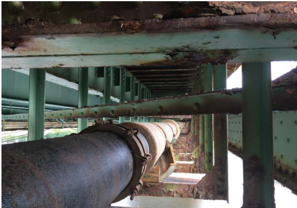
Photo #48: General view of lateral bracing spanning between utility supports in span 1 & 2 (8/1/16)
