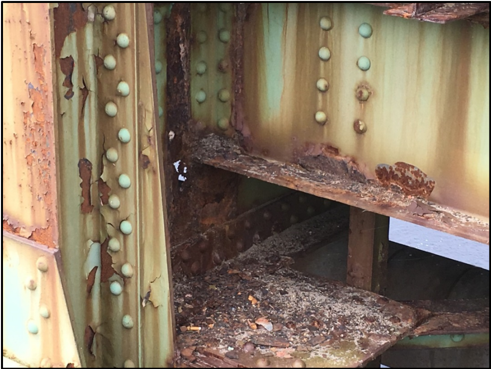
Photo A1 – Floorbeam 7, Roadway Truss @ Stringer 8 (Exterior)
