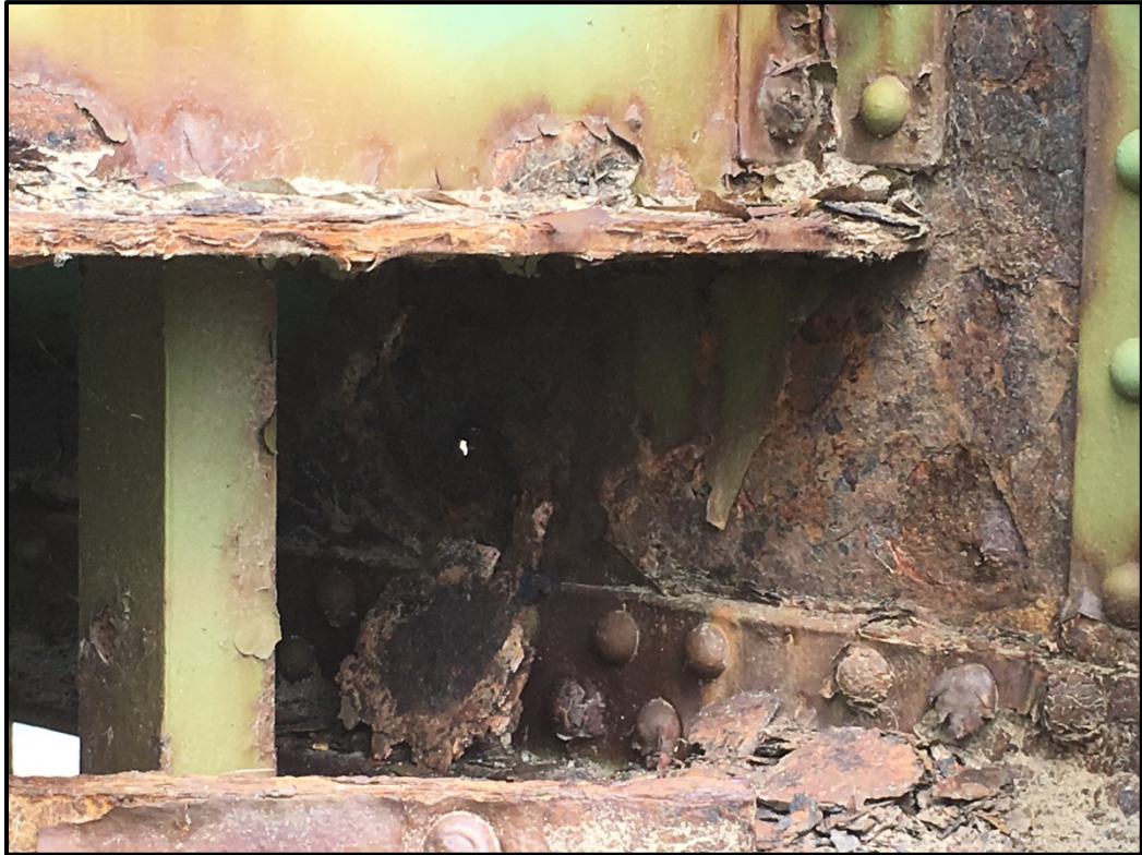
Photo A3 – Floorbeam 2, Roadway Truss @ Stringer 8 (Exterior)
