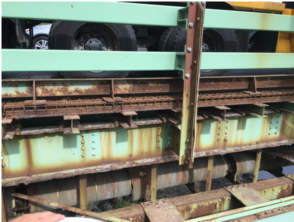
Photo #4: General view of the superstructure section (8/1/16)
