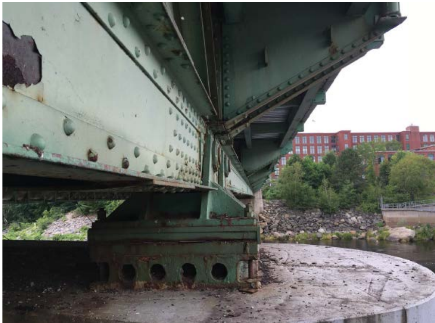
Photo #56: Typical view of the bearings at pier 1 (8/1/16)
