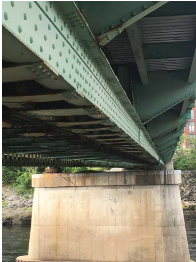
Photo #3: General view of the underside of the sidewalk side of the bridge (western side, Span 2 looking south) (8/1/16)
